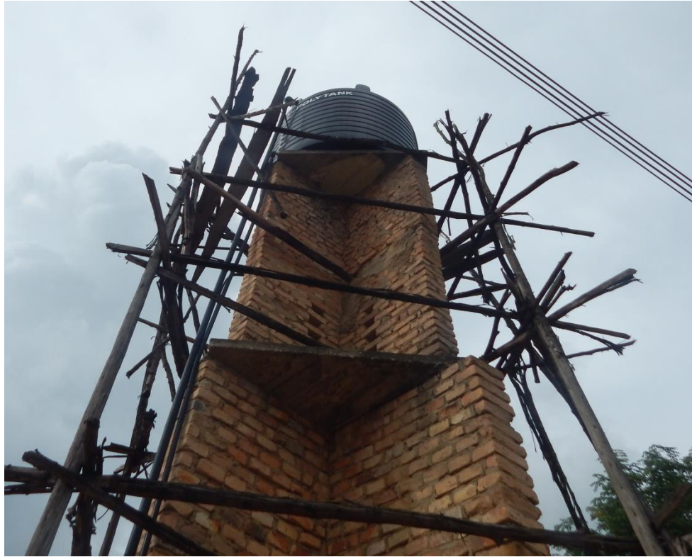
Figure 4: 5,000 L tank on 8 m water tower
